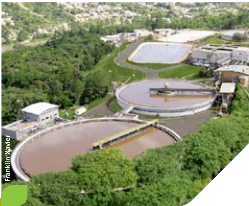
Effluent Treatment Plant in Monte Alegre
